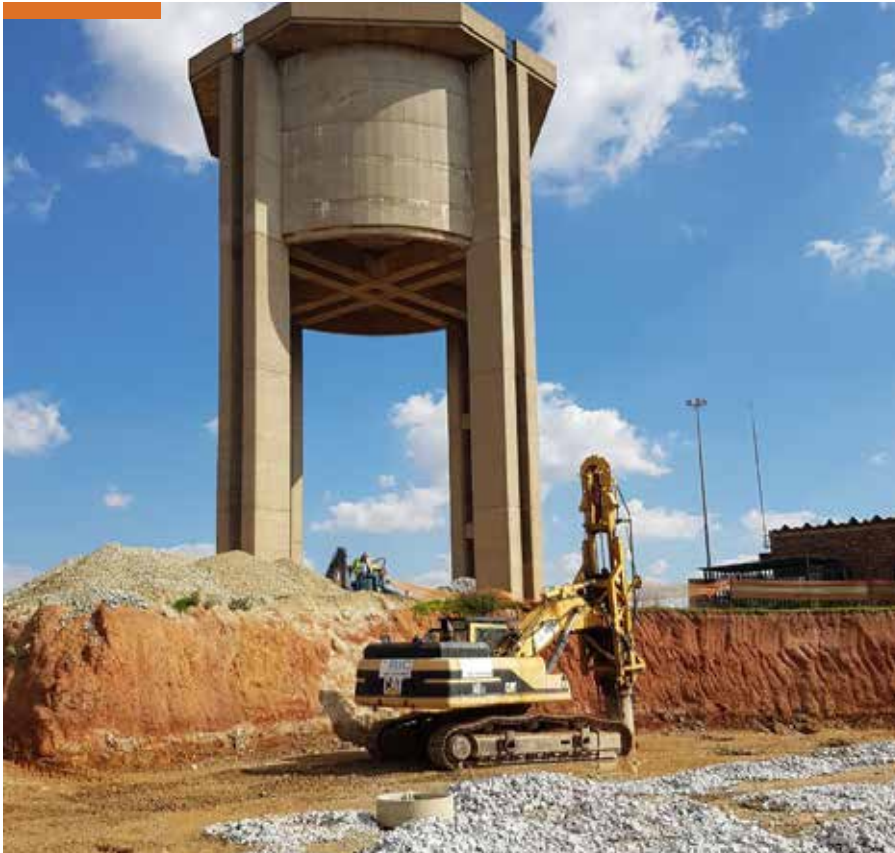
Rapid impact compaction at Zulu Xhosa Reservoir
